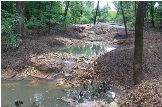
**Rushing stormwater had eroded** a stream called Milkhouse Run in Washington, D.C.'s Rock Creek Park, exposing a sewer pipe and carrying soil downstream (above). In 2011, engineers reworked the stream channel, installing shallow pools, weirs, and native vegetation to slow water flow and reduce erosion (below). This type of restoration design is called a regenerative stormwater conveyance. PHOTOGRAPHS, BIOHABITATS INC.
