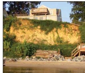
**A long line of gabions** (metal cages containing large rocks) was installed in fall 2013 to protect this cliff base in Scientists' Cliffs. Erosion along the length of the cliffs threatens to overtake several homes, dumping them into the surf. PHOTOGRAPHS: LEFT, DANIEL STRAIN; RIGHT, DAVID BROWNLEE
