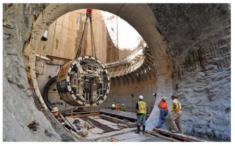
Workers sink a shaft at street level in a dense neighborhood at 1st and V Streets, N.W., in Washington (right) as part of a tunnel-building project below. Pieces of a giant tunnel-boring machine are lowered (above) and assembled underground. The machine bores space for a tunnel 23 feet wide to store a mix of stormwater runoff and sewage to improve water quality. PHOTOGRAPHS, DC WATER
