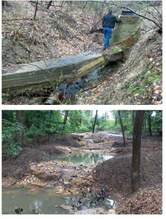
**Rushing stormwater had eroded** a stream called Milkhouse Run in Washington, D.C.'s Rock Creek Park, exposing a sewer pipe and carrying soil downstream (above). In 2011, engineers reworked the stream channel, installing shallow pools, weirs, and native vegetation to slow water flow and reduce erosion (below). This type of restoration design is called a regenerative stormwater conveyance. PHOTOGRAPHS, BIOHABITATS INC.
