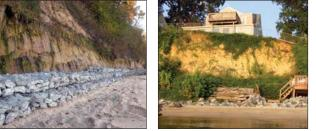
**A long line of gabions** (metal cages containing large rocks) was installed in fall 2013 to protect this cliff base in Scientists' Cliffs. Erosion along the length of the cliffs threatens to overtake several homes, dumping them into the surf. PHOTOGRAPHS: LEFT, DANIEL STRAIN; RIGHT, DAVID BROWNLEE
