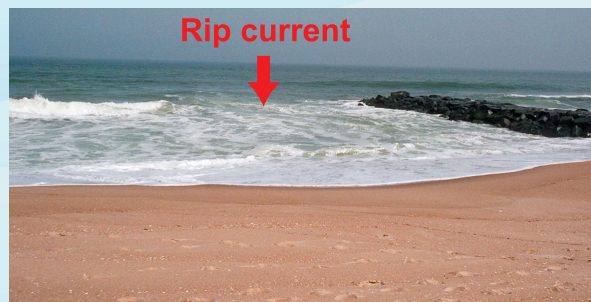
Rip currents often form near coastal structures.
